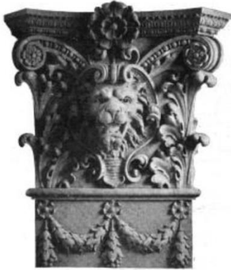
TERRA-COTTA CAP, OFFICE BUILDING, 78 FIFTH AVENUE, NEW YORK CITY. Albert Wagner, Architect. Made by White Brick and Terra-Cotta Company.
