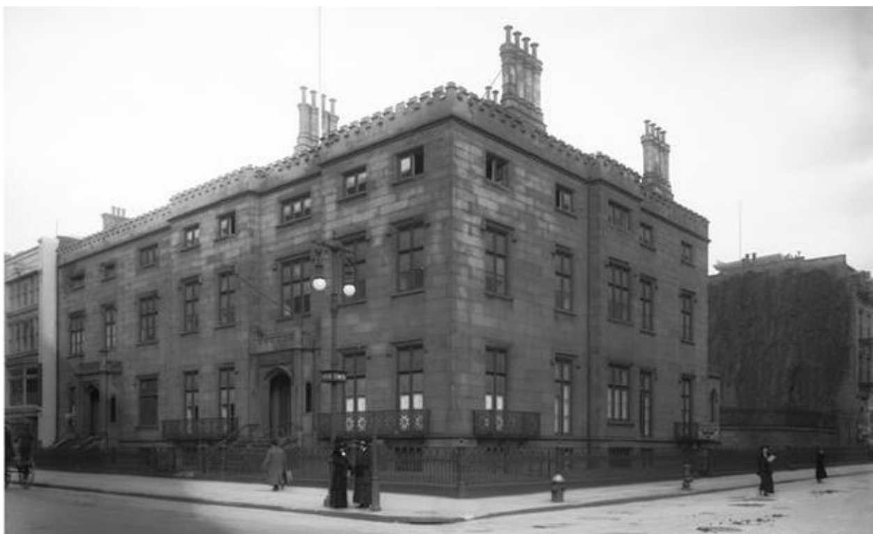
The former James Lenox's Mansion, 53-55 Fifth Avenue, with 57 Fifth Avenue visible at far left, ca. 1911, just prior to demolition. Wurts. Bros, MCNY.
